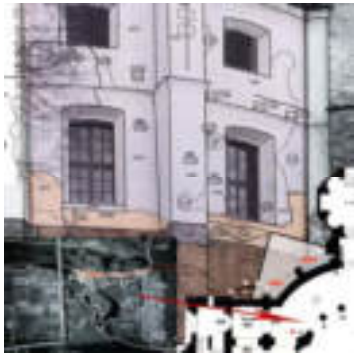
Figure 3. The various phases of construction (roman, late-ancient, medium age, modern age, and restoration) georeferenced thanks to interdisciplinary analyses (C14 samples, thermoluminescence, archaeometric, and so on) highlighted recovered bricks, dated the mortar between the bricks, etc
