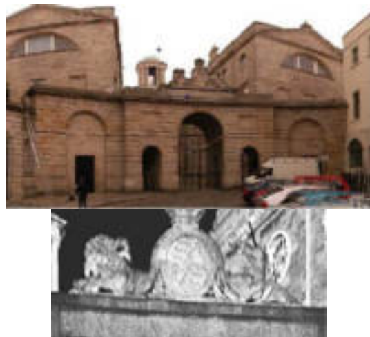
Figure 8. Image and point cloud of stone carving at bottom of street, the 3d point cloud is ideal for capturing sculpting and carving.
