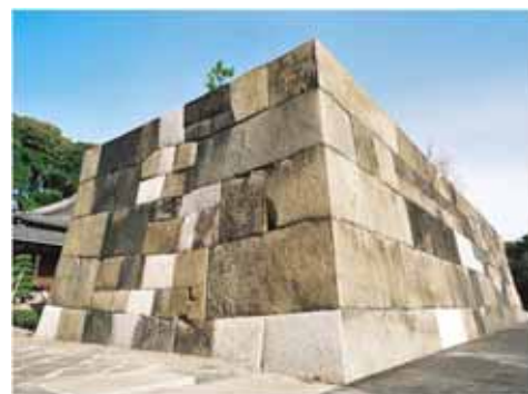
Figure 2: After the restoration
