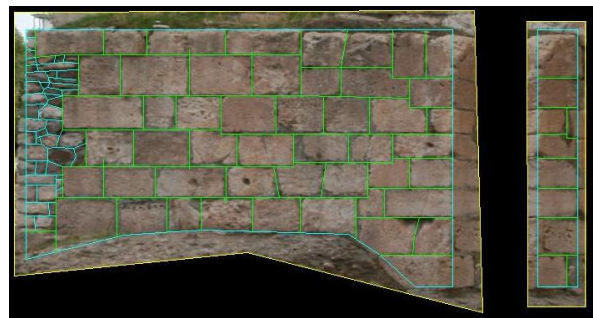
Figure 5: Vectorising of joints between the stones
