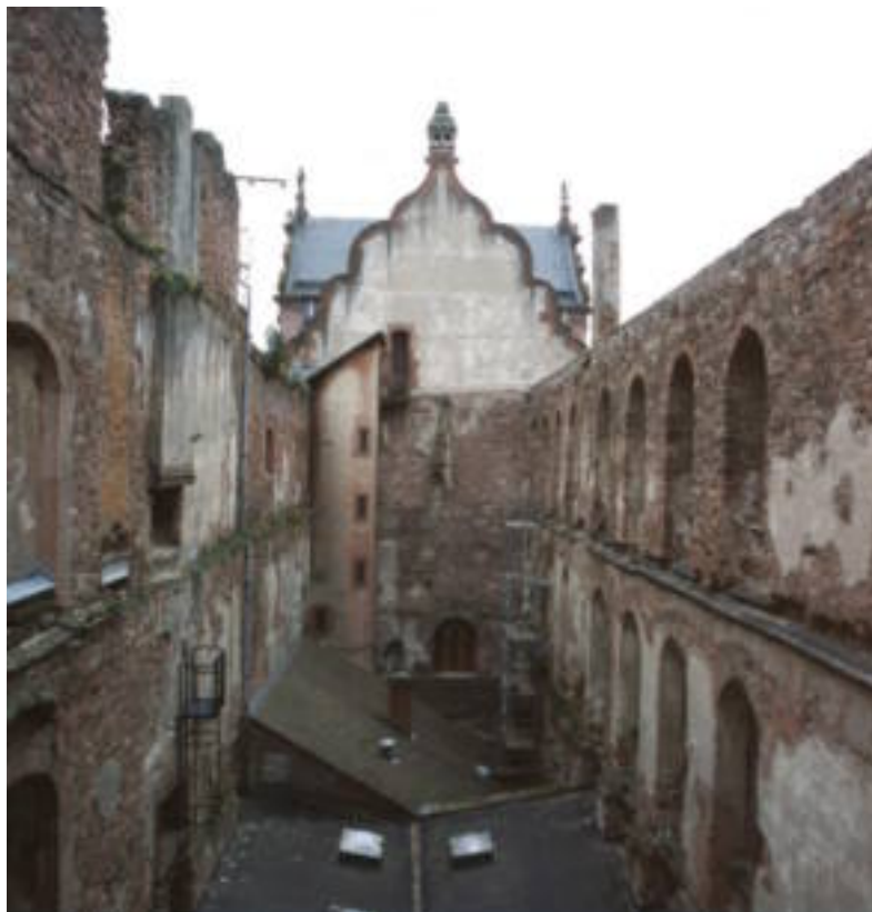
Figure 1: The interior view of the renaissance building “Gläserner Saalbau”.
