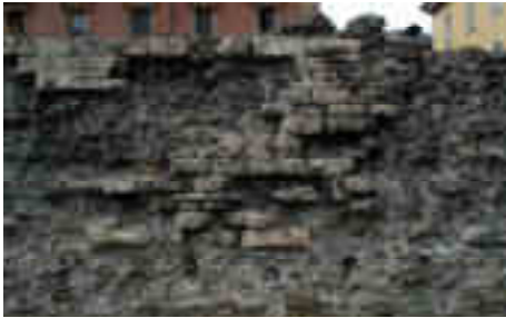
Figure 2. Portion of wall belonging to the Aosta wall perimeter that delineates its conformation
