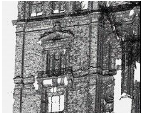
Figure 5: Incomplete and striated information linked to balconies and ornamental details in the façade of the City Hall
