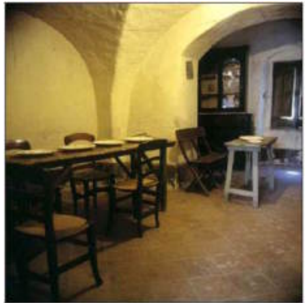
Image 11: Barrel vaults, cross vaults characterize the rooms on the ground floor
