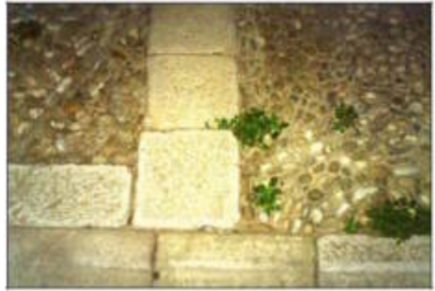
Image 10: The inner rooms paved in riverbed stones
