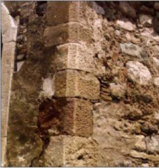
Image 8: Sandstone masonry made with irregular blocks
