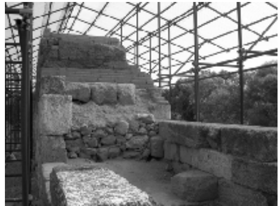
Figure 11. Gela: masonry section ( emplekton )
