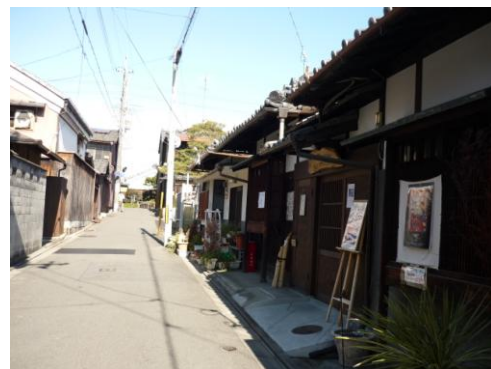
Figure 7. Concatenated machiya in good condition (Demizu district)
