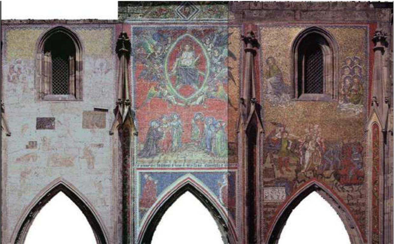
**Figure 5:** Rectified images of the facade, showing its state before conservation (left ), after treatment (center), and after gilding (right). Jaroslav Zastoupil.
