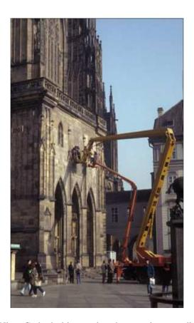
**Figure 3:** Conservators at St. Vitus Cathedral inspecting the mosaic, recording conditions on transparencies overlaid on rectified photographs of the facade. Photo: Dusan Stulik.
