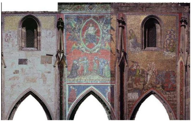
**Figure 5:** Rectified images of the facade, showing its state before conservation (left ), after treatment (center), and after gilding (right). Jaroslav Zastoupil.
