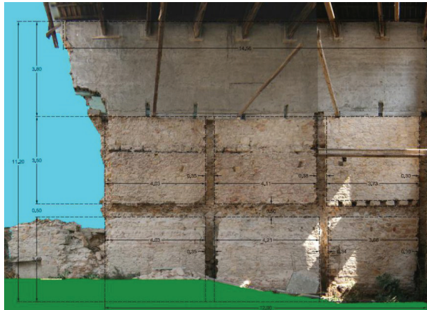
Figure 11. Necessary information about the eastern masonry obtained by the orthomosaic (left) and the view of the eastern masonry after the completion of the support (right)
