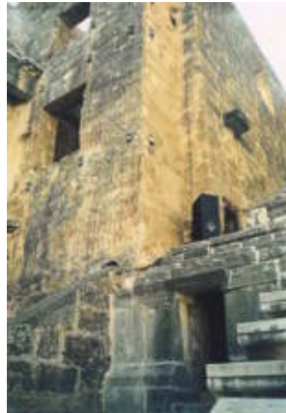
Figure 4. Northern Side Wall and Seljukian Plaster on Analemma wall
