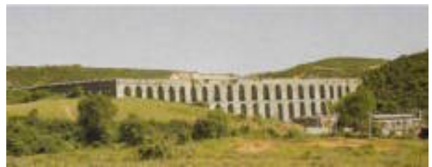
Figure 6. The Kovukkemer aqueduct
