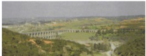
Figure 5. The Kovukkemer aqueduct
