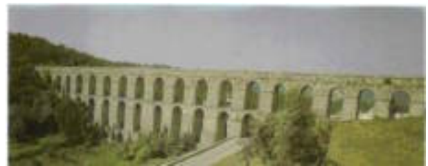
Figure 7. Main façade of the Kovukkemer aqueduct
