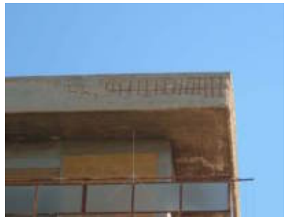
Figure 16. Particular of the wall of the attic in situated building to Villaseta – AG, separation of the plaster of covering of the wall of the attic.; deficiency of abutement stone; machines of humidity and manifestations of the “effluorescenza” in the intrados of the floor of the covering terrace
