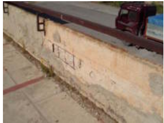
Figure 15. Villaseta – AG, supporting wall - presence of the humidity of the reclimbing and separations of the plaster for rainwater infiltration
