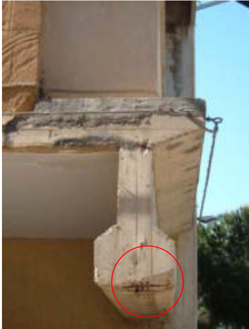
Figure 13. Particular of the degraded prospect in situated building in Villaseta – AG
