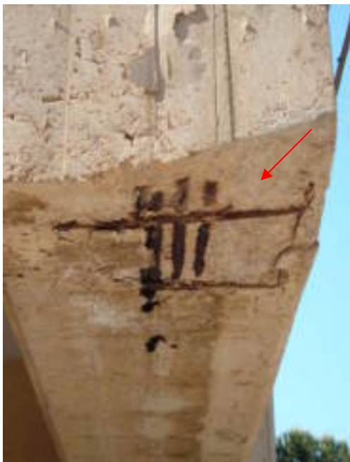
Figure 14. Particular in prospect of situated building in Villaseta – AG, degradation of cls, the oxidized armor
