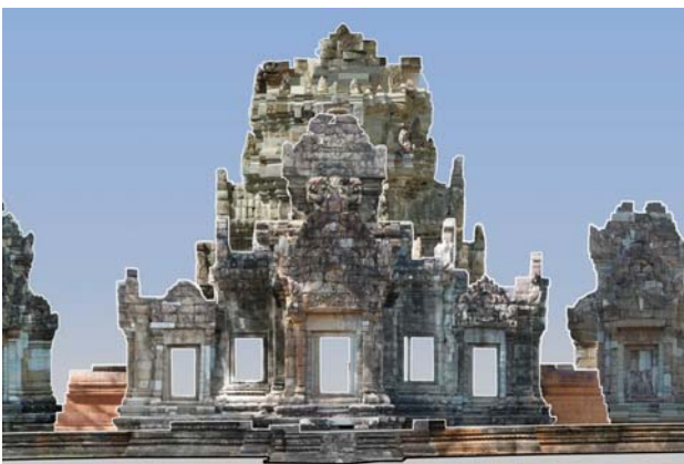
Figure 13. As-bulit survey of Chau Say Tevoda, Angkor Monuments, Cambodia (after restoration)
