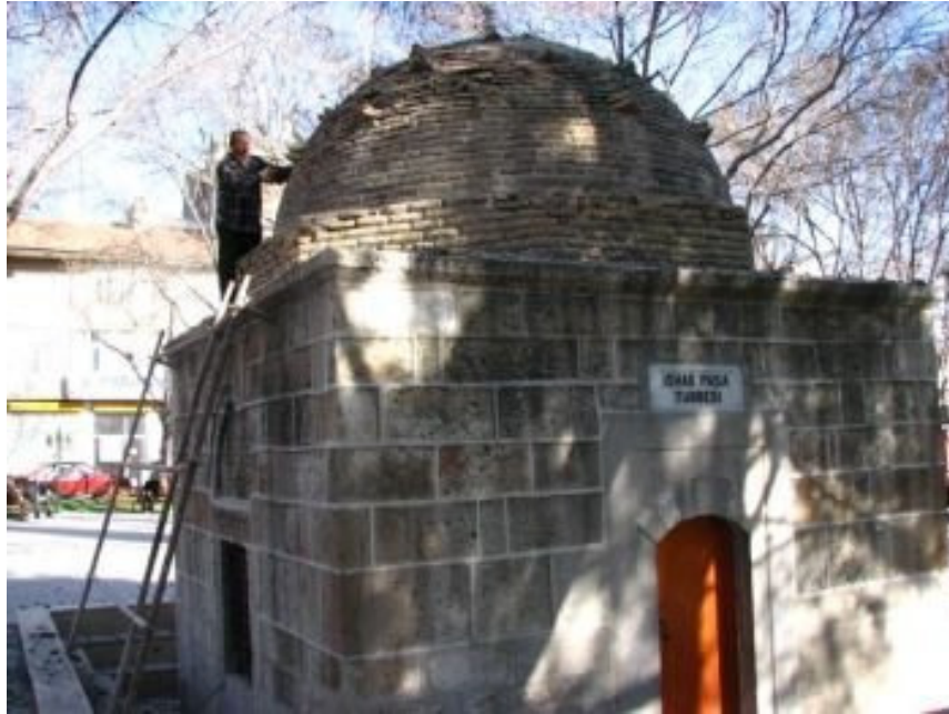
Figure 2. The restoration works on Tomb
