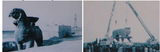
Figure 4. hanging and moving of Cangzhou iron Lion (1984)
