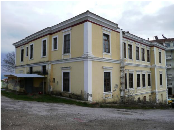
Figure 6 Old prefecture of Kilkis (view from west)
