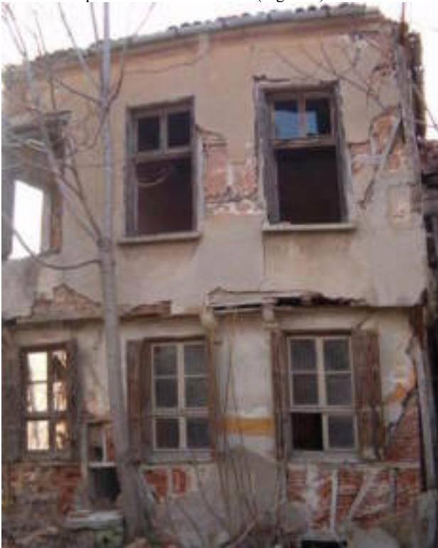
Figure 4. Decay in the timber frame structure
