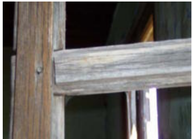
Figure 2. Splitting along the connection points in the casements and surface cracking
