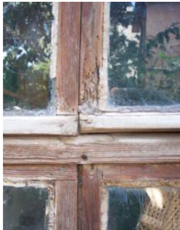
Figure 3. Insect damage to the window casements and textural damage
