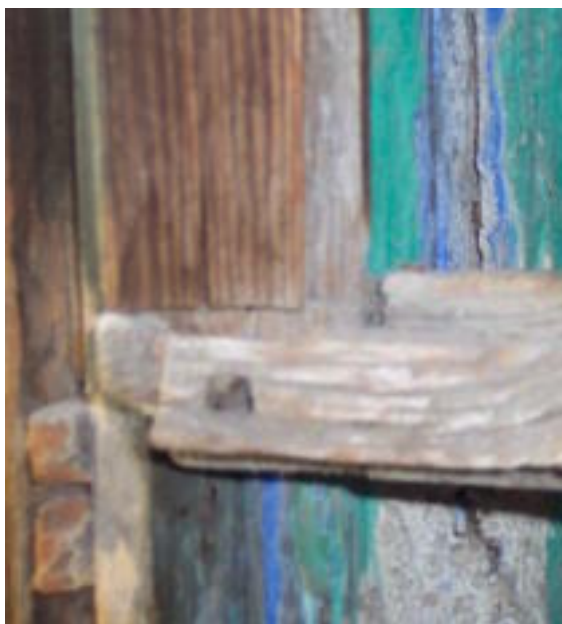
Figure 1. Wear and tear on the window casements and jamb.
