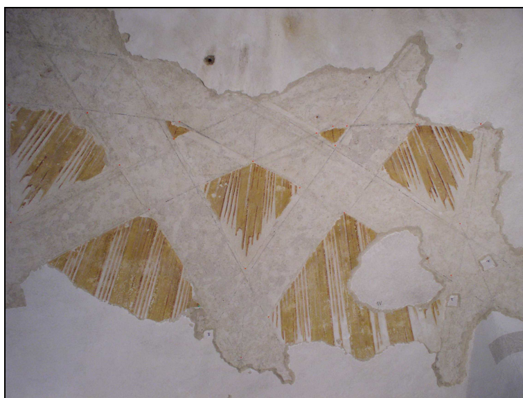
Figure 2: Part of the foundations of original stucco work from the period of Santini. (Photo: Jaroslav Zastoupil)
