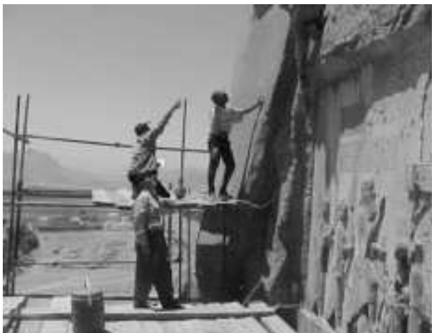
Figure 6: preparation of the work
